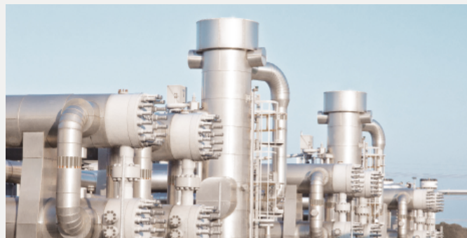
Pict. 2: PtL factory 6MW / 200 l/h
